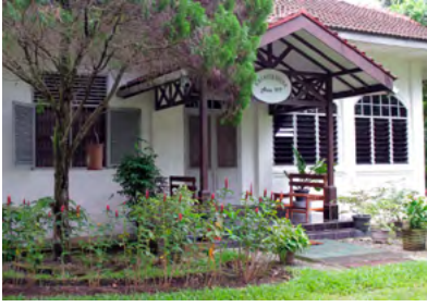
📷 Manager's bungalow at Tanah Besih Estate, dating from 1917.
