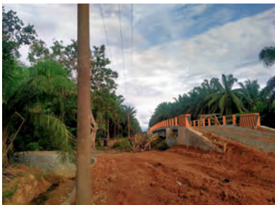
📷 New bridge erected at the Seunagan estate, which will be used for many years ahead by communities and the plantation alike.
