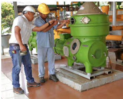
📷 Preventive maintenance, to keep a safe workplace.
