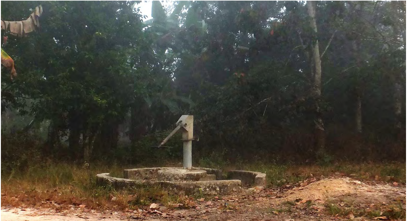
Unused SRC hand pump in Gorbor
