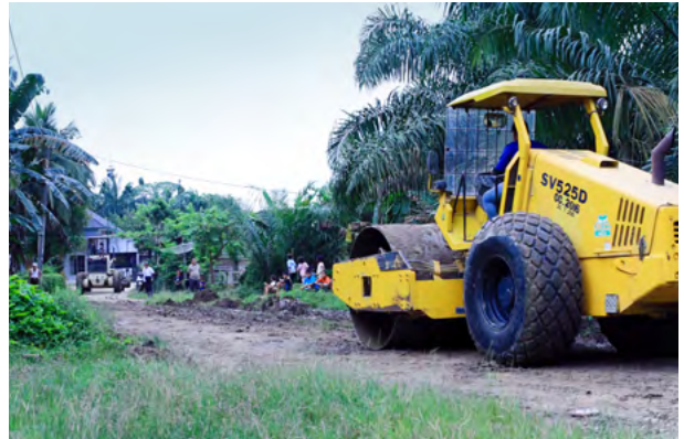
📷 Heavy equipment assistance on some of our communities' roads.
