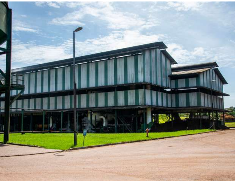
△ Oil mill, Mbambou, Socapalm, Cameroon
