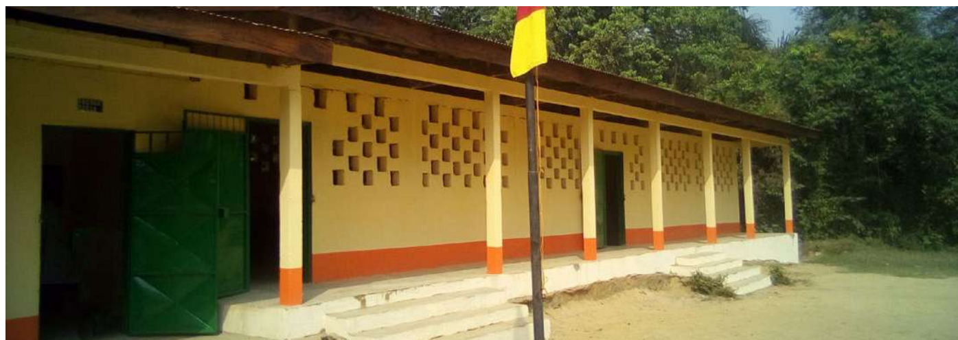
△ Rehabilitation of Songueland Public School, Safacam, Cameroon
