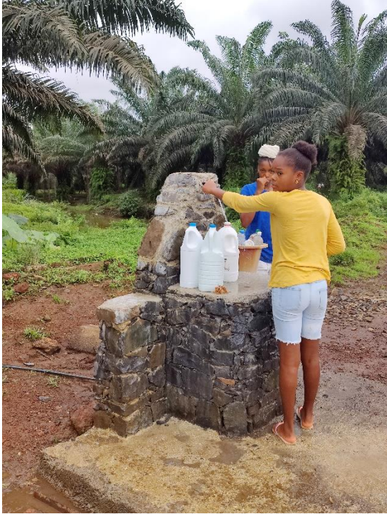
Figure 23: Water well construction in Emolve
